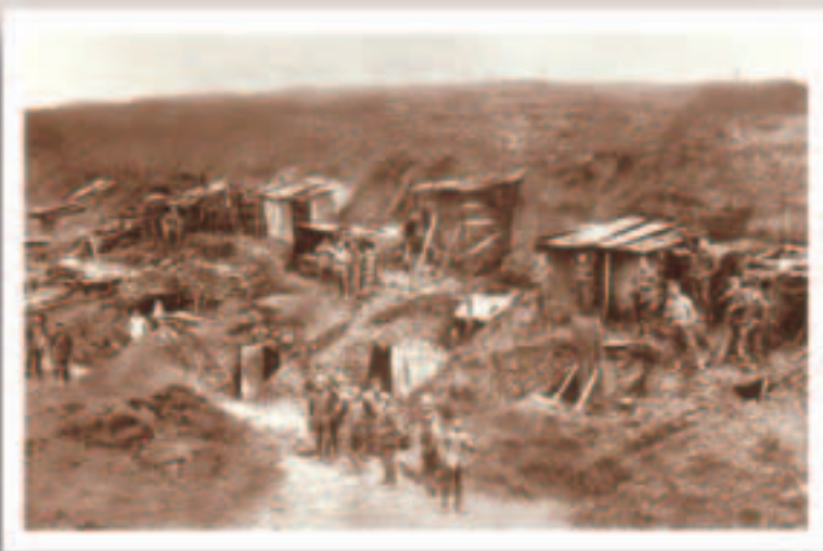
German dug-outs. German quarters behind the line were little different from those of Canadians —, but because they usually held the higher ground, their front line dug-outs were usually deeper, better-built, and better drained. [DND DHist-8]
